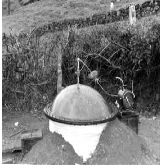
Figure 4: Localized (self-sufficient and contained) anaerobic methane digester 14
