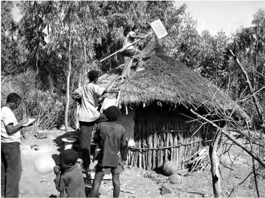
Installation of off-grid solar energy by Solar Energy Foundation. 28
