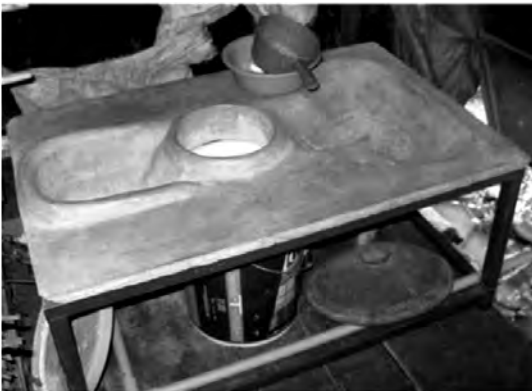
Figure 3: Locally made urination/defecation separation toilet (household scale) 13
