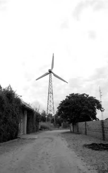
150kW wind turbine, in Batakunku, The Gambia. 34
