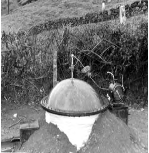
Figure 4: Localized (self-sufficient and contained) anaerobic methane digester 14
