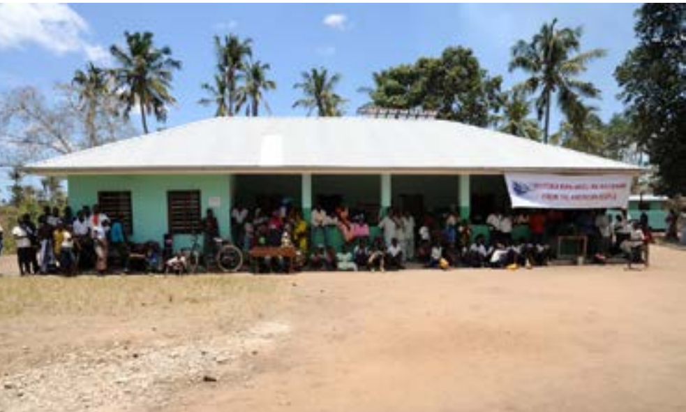
Figure 2. A healthcare clinic in Tanzania. The clinic was renovated in 2009, as it previously had no electricity, no water, and no toilets. Medical waste was burned outside the clinic, and the nearest water source was five miles away 6 .
