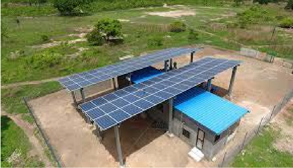
Off-Grid solar energy at Wayo Atingagorme, a remote Island in Ghana. Photo by: John Deyegbe/Resolution Ltd.
